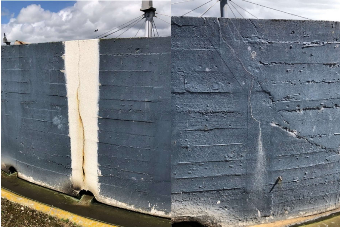
Figure 1: Trickling filter showing structural condition
